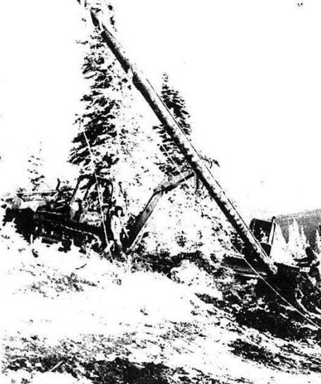
ERECTING a power pole on a slope, at 1,855 metres (6,100 feet) above sea level, can be tricky business as work crews on Silver Star Mountain have found out. The first
