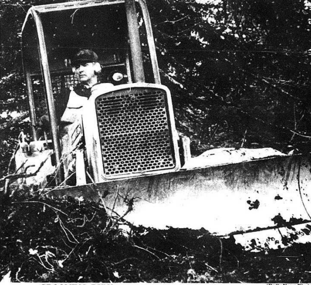
GROOMING RUNS (Daily News Photo) One of the main projects this year at Silver Star Ski Area has been grooming. Operations Manager Walt Keckalo and his crew have improved the Whiskey Jack, Blue Chair, Far Out, and Way Out runs. The grooming process includes stump removal, widening, and grass planting.
