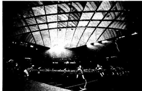
MODERN ART? More like the setting for a modern art — professional football. Geometric-patterned dome, above, covers the new Pontiac, Mich., Stadium, home of the Detroit Lions. Below, the 400,000 square foot air-supported dome is of Teflon-coated Fiberglass fabric, erected by Construction Services Division of Owens-Corning Fiberglass Corp.
